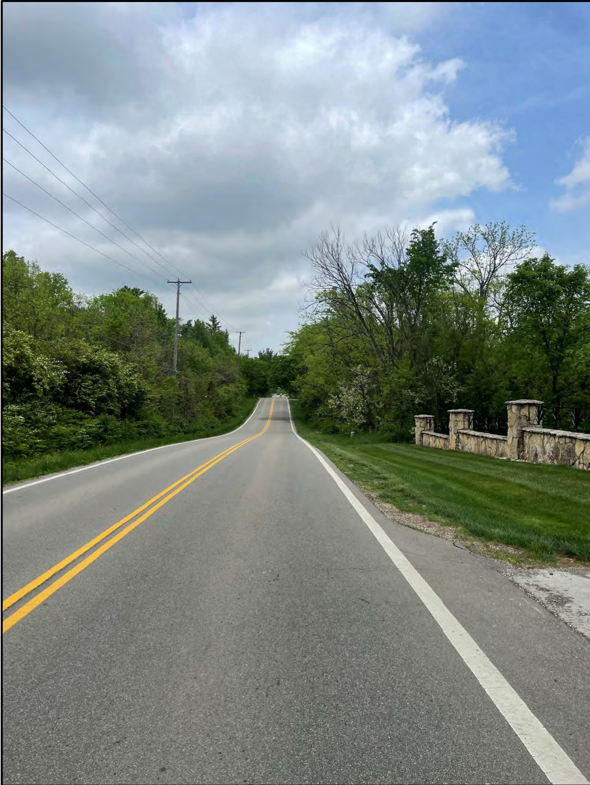
Photo 2 – Sight Distance, 665' North of Proposed Access
